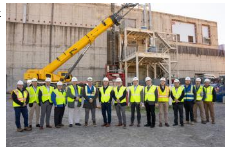
Under Secretary for Nuclear Security and NNSA Administrator Brandon Williams viewed progress at the Savannah River Plutonium Processing Facility (SRPPF) with senior federal and contract leadership.
