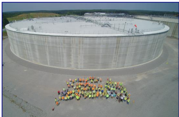
Saltstone Disposal Unit 8 project team members stand in front of the newest mega-size disposal unit completed at the Savannah River Site.
