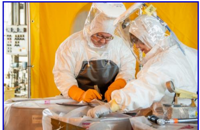
H Canyon Outside Facilities Operator Andrew Pratt (left) and H Canyon Outside Facilities Radiological Control Operator Wanda Patterson load drums of depleted uranium solution that was prepared for addition to ABD material. The depleted uranium addition helps meet the safety limits for each material transfer from H Canyon to DWPF.
