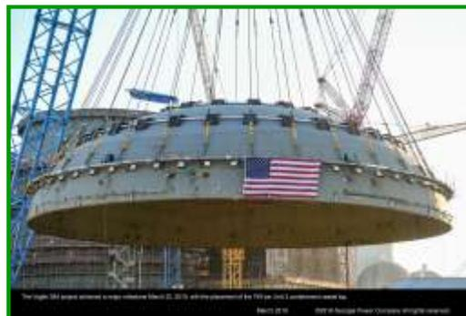
The containment vessel is a high-integrity steel structure that houses critical plant components. The top head is 130 feet in diameter, 37 feet tall, and weighs nearly 1.5 million pounds, more than two fully loaded jumbo jets. It's comprised of 58 large plates, welded together, each more than an inch and a half thick.
