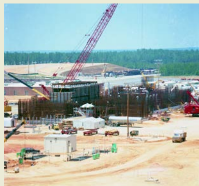
Construction of the Defense Waste Processing Facility
