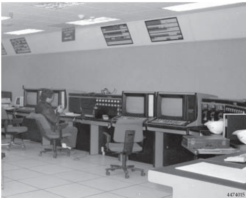
Figure 4. Modern control room for replacement precipitators
